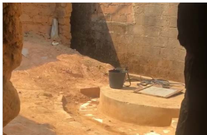
Remnants of the original church building that survived the war.
